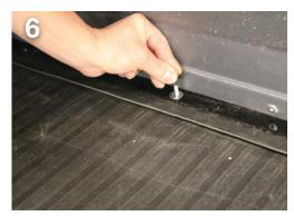
Insert the partition and loosely secure it to the floor using 1 ½" screws (**E**), washers (**C**), and split washers (**D**).
