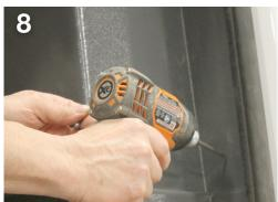
Using self-drilling screws (**F**) in the predrilled holes, loosely secure the rest of the partition. When properly positioned, tighten all bolts.
