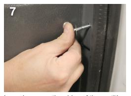
Loosely secure the sides of the partition with the 2" screws (**G**), washers (**C**), and split washers (**D**).
