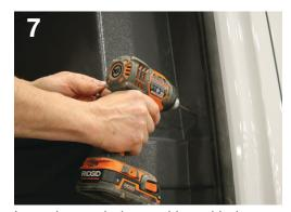
Loosely attach the partition with the 1 ½" Philip screws (**D**), flat washers (**B**), and split washers (**C**) to all areas where plus nuts were installed in step 5.
