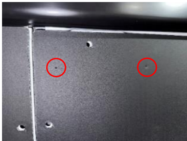
Holes marked for drilling
