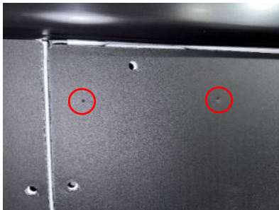
Holes marked for drilling
